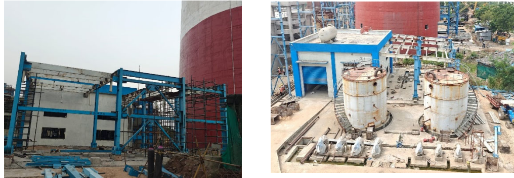
ECW/ ACW Building
