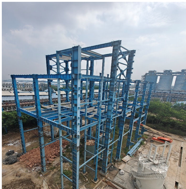
Gypsum Dewatering Building – Structure erection (Tier 3)
