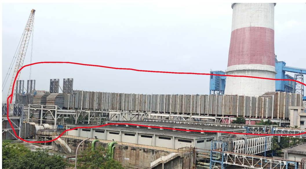
Duct U#4 & U#5 – Major ducting work completed after Mar'25 (Approx 700 MT)
