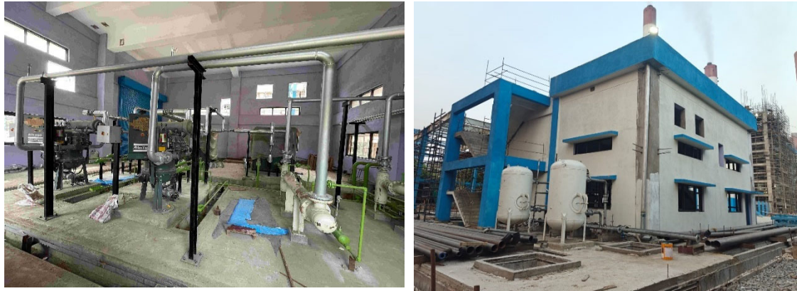
Compressor House - Equipment and piping Made ready After June'25
