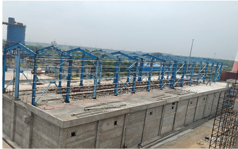
Gypsum Shed – Finishing and Structure erection activities after June'25
